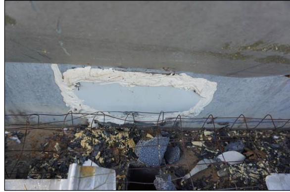
Figure 6. Metal plate over inside face of scupper opening
