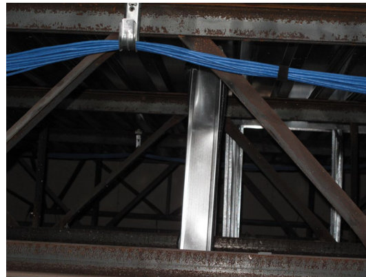
Figure 6: Buckled cold-formed steel stud
