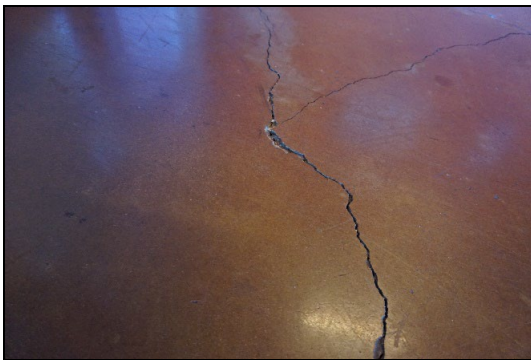
Figure 9: Fractured concrete slab-on-grade exhibiting vertical offsets
