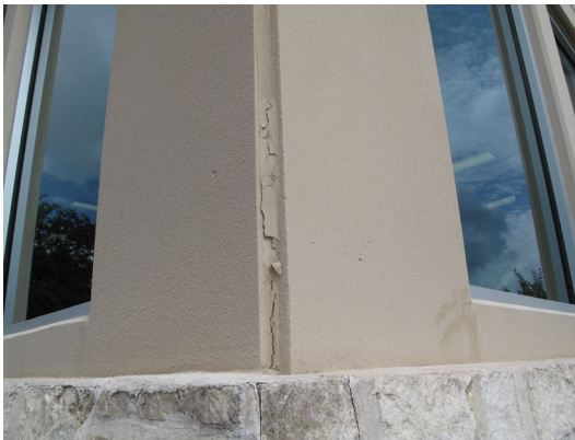
Figure 5: Tilt-up wall panel joint separations
