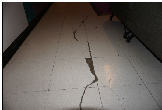
Figure 10: Fractured tile floor; visibly sloping floor
