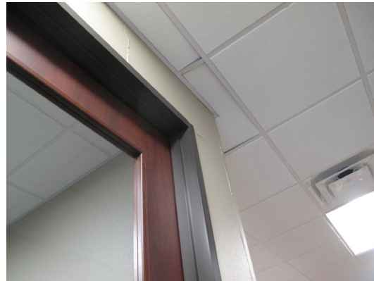
Figure 4: Displaced ceiling panels
