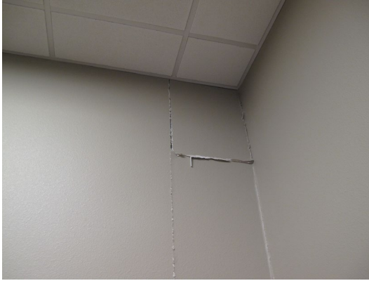
Figure 1: Gypsum board separations and fractures
