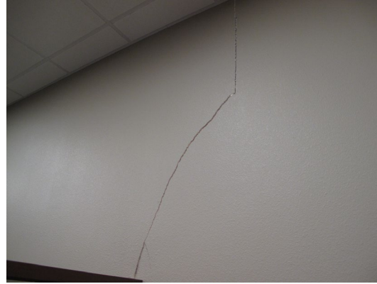
Figure 2: Gypsum board separation and fracture
