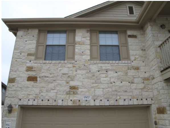
Figure 6: Overview of typical survey area at stone masonry veneer.
