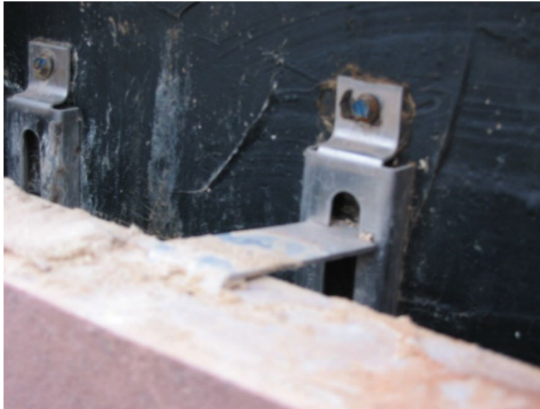
Figure 12. Tie installed such that it restrains vertical movement of the veneer.
