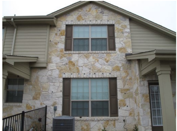
Figure 7: Overview of typical survey area at stone masonry veneer.
