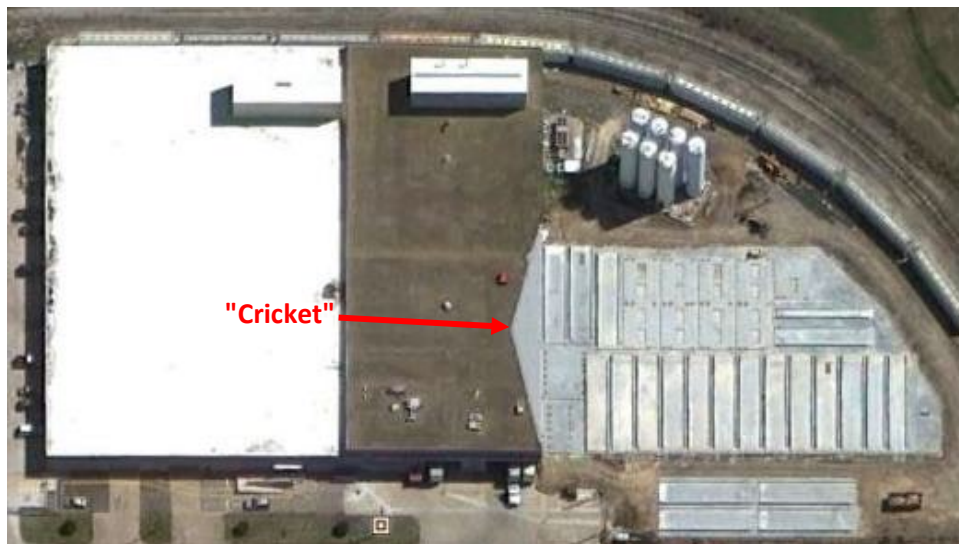
Figure 2. A view of the facility during the construction of the new building addition. Note the drainage "cricket" installed along the drainage edge.
