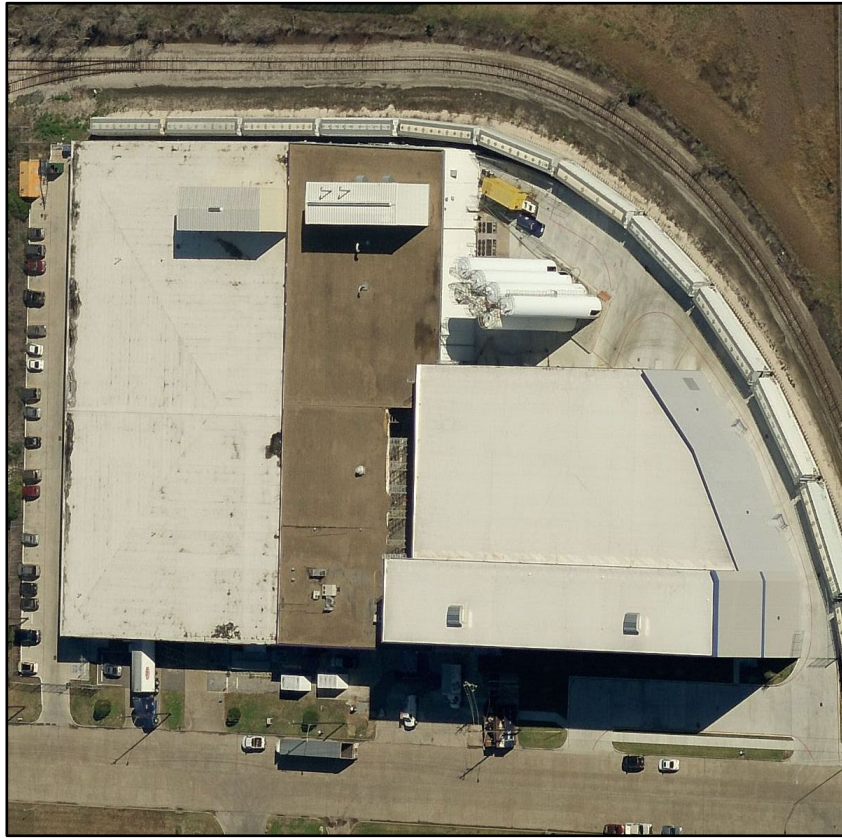
Figure 3. View of the facility with the new building addition and the collapse area.
