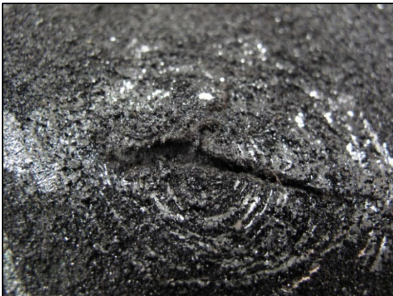
Figure 7: Interply bitumen disturbance with felt ply rupture evident, from impact F-2 (light pressure applied from below)
