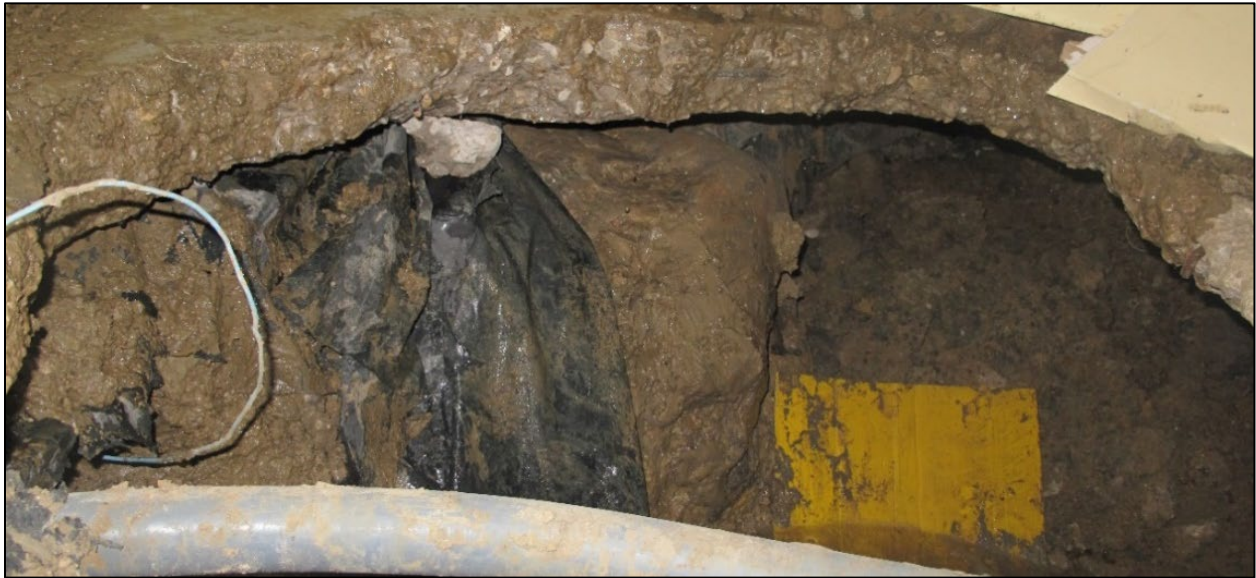
Figure 6: Visible void below the concrete slab adjacent to the fire riser
