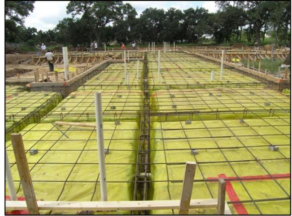
**Figure 16:** Vapor barrier at the slab portions and grade beams of the foundation (image included with permission).
