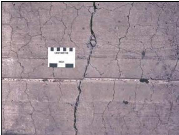
**Figure 1:** Traditional ASR map cracking.
