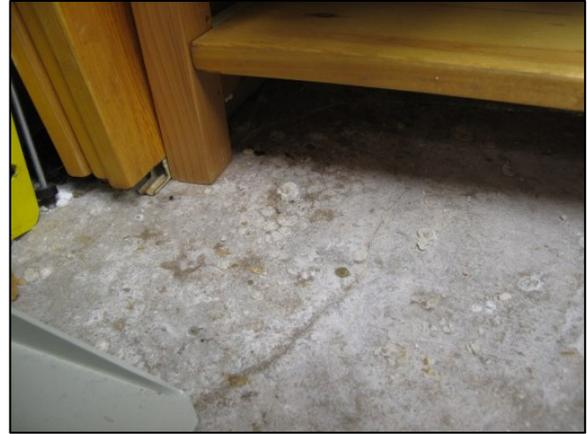
**Figure 10:** Close-up view of gel exudations and surrounding white residue.
