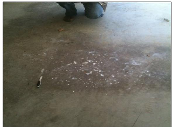
**Figure 18:** Close-up view of white residue at concrete slab surface (image included with permission).
