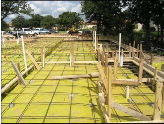
**Figure 15:** Vapor barrier at the slab portions of the foundation (image included with permission).
