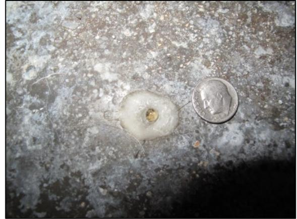
**Figure 6:** Close-up view of gel exudations and surrounding white residue.
