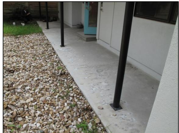
**Figure 4:** Gel exudations at concrete slab surface at back patio – note the checkered pattern.
