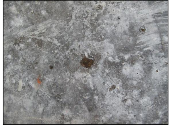
**Figure 8:** Close-up view of new gel formation with no hard outer layer.
