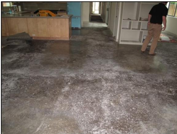
**Figure 3:** Gel exudations at concrete slab surface at interior – note the checkered pattern.
