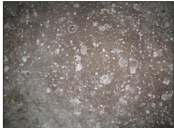
**Figure 2:** Gel exudations and white residue from NSASR at concrete slab surface.
