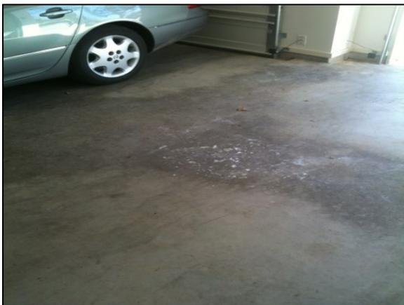
**Figure 17:** White residue and discoloration at concrete slab surface – note the checkered pattern (image included with permission).
