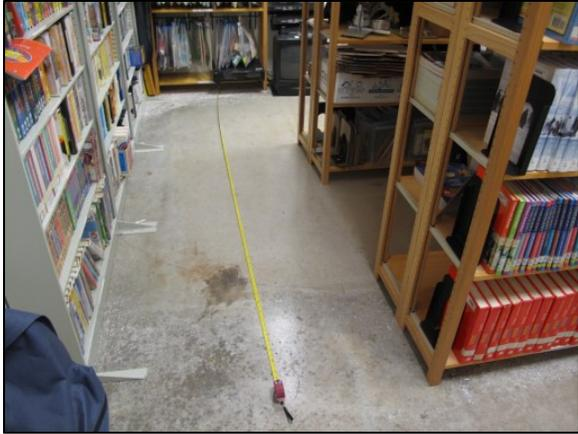
**Figure 9:** Gel exudations at concrete slab surface – note the checkered pattern.
