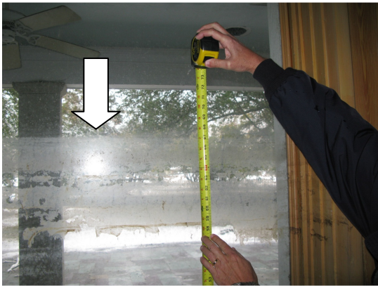
Figure 5: Residential Living Room Window
