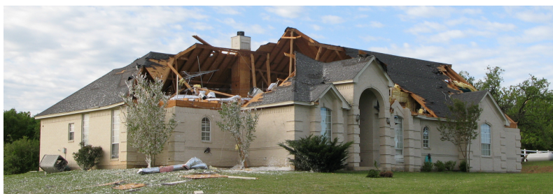
Figure 7. Condition of structure
