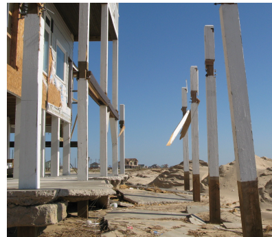
Figure 10. Missing/displaced framing
