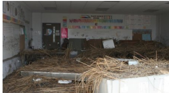
Figure 3. Papers still intact at interior
