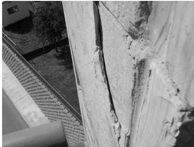
Figure 3. View of stone veneer – note vertical orientation of the grain.
