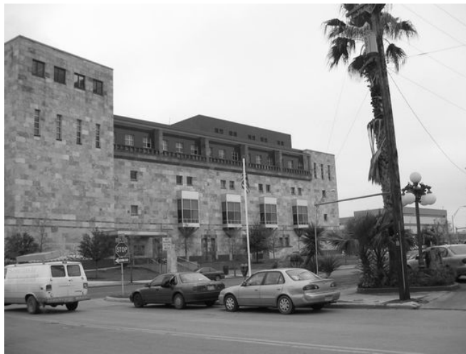
Figure 1. General view of Building A exterior.
