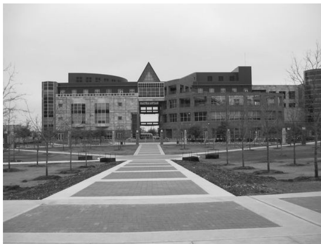
Figure 2. General view of Building B exterior.
