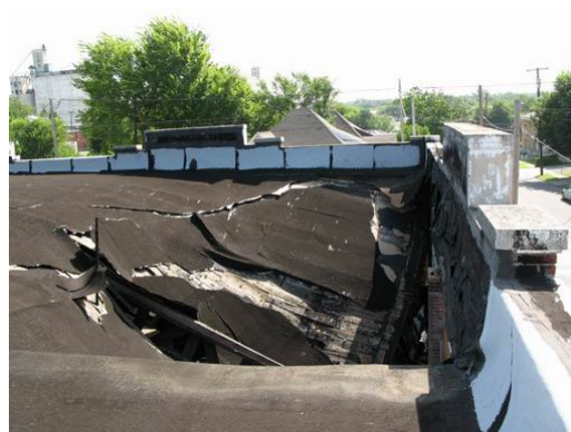
Figure 12. Partial roof collapse.
