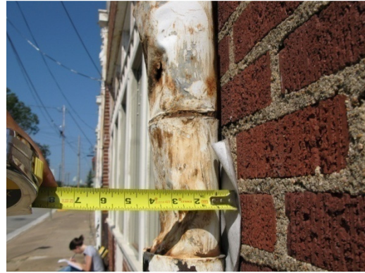
Figure 14. Reduction in downspout cross-section.
