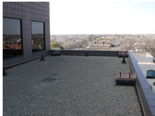
Figure 9. Ballasted built-up roof.
