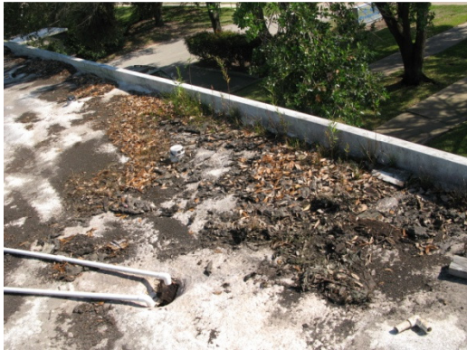
Figure 4. Debris build-up at roof.
