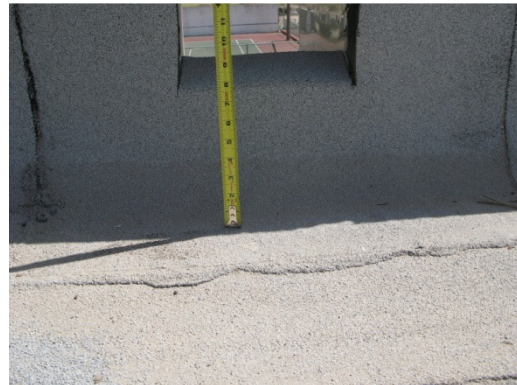
Figure 3. Additional scupper located 7" above the roof surface.
