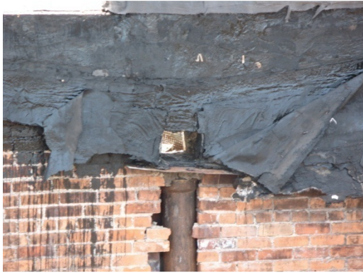
Figure 13. Modified drainage – scupper above sealed-over drain.
