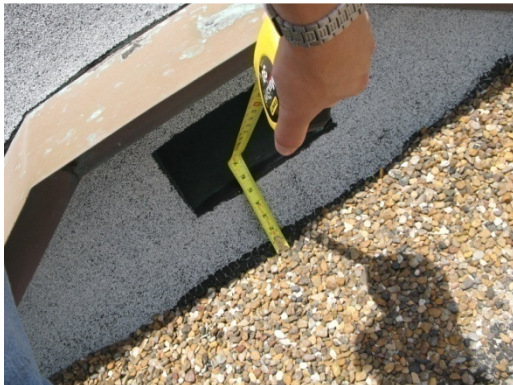
Figure 2. Scupper is located approximately 5" above the roof surface.
