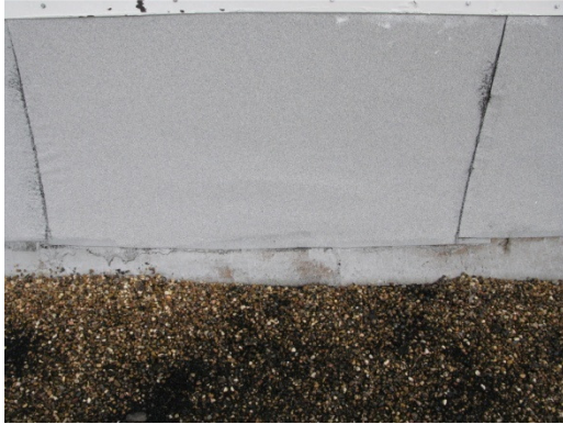
Figure 6. Patched over overflow scupper.
