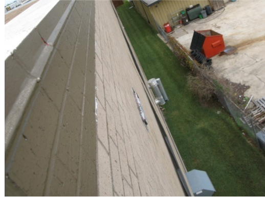
Figure 7. Non-functional scupper viewed from exterior.
