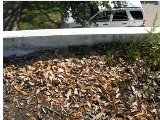
Figure 5. Debris build-up around scupper.
