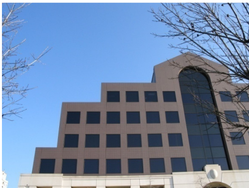
Figure 8. Recessed cascading roofs.
