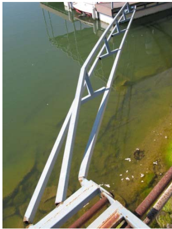
Figure 3. Failed stiff-arm.
