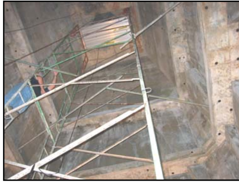
Figure 3. Dome interior (looking up).
