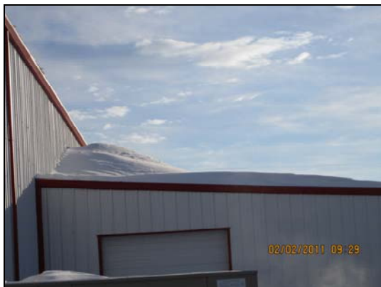
Figure 4: Snowdrift geometry/height at southern lower roof
