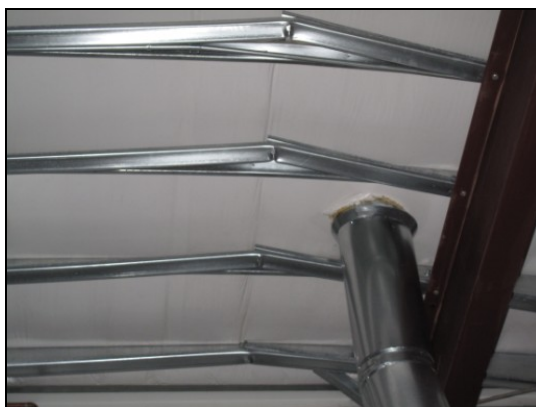
Figure 6: Failed Z-purlins
