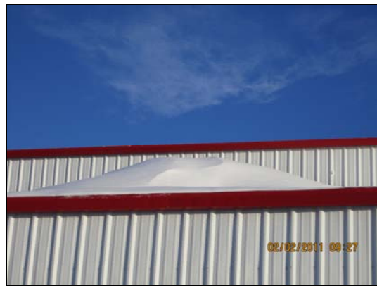
Figure 3: Snowdrift geometry/height at southern lower roof
