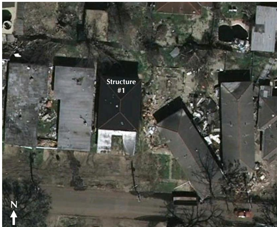
Figure 6: Structure #1 & Adjacent Properties
