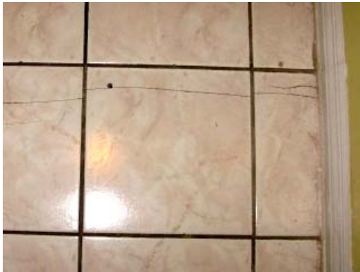
Figure 7: Reflective fracture in tile.
