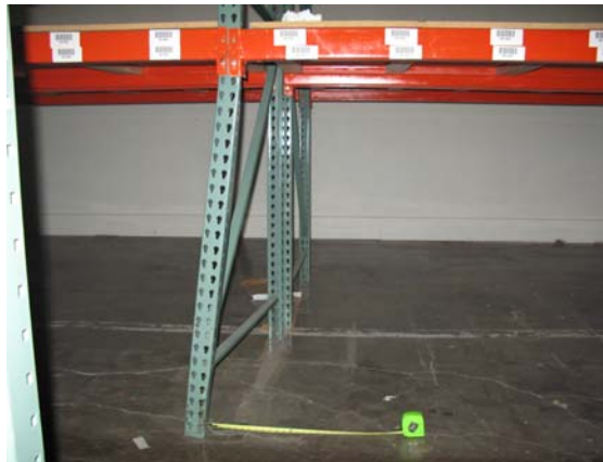
Figure 5: Out-of-plumb Column
