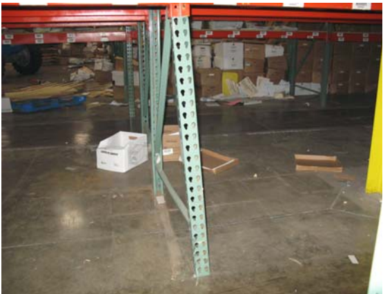
Figure 4: Out-of-plumb Column
