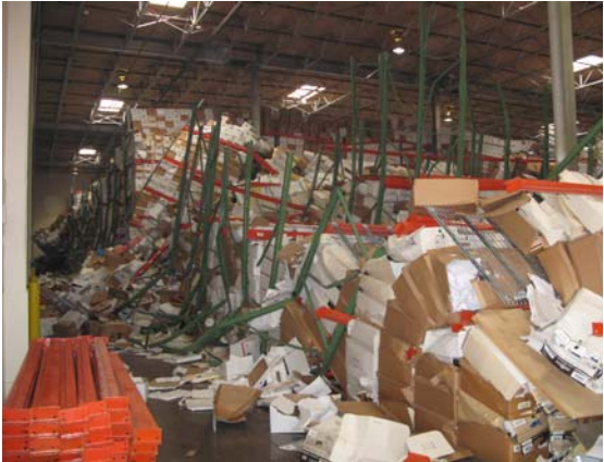
Figure 1: Collapsed Storage Racks
