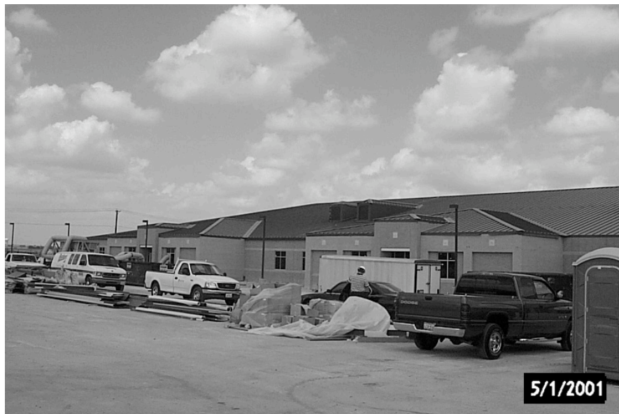
Figure 6. School structure. Note metal roofing.
