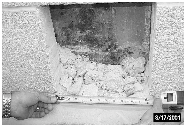
Figure 4. Typical mortar droppings at removed block B2.
