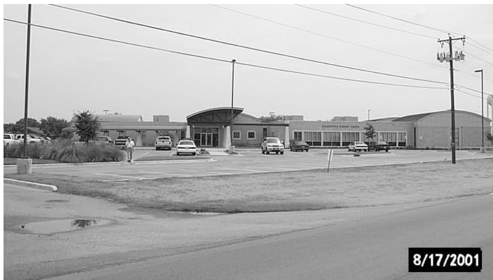
Figure 3. Front elevation of structure.
