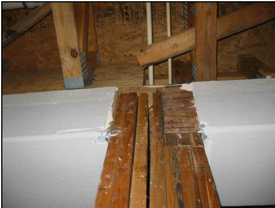
Figure 4. Top of columns. Distance between columns same as at base.
