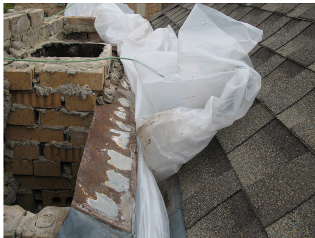
Figure 4. Full Penetration of Metal Flashing
