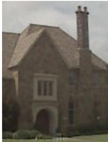
Figure 5. Pre-storm Chimney at Case Study B (Google Maps Street View)
