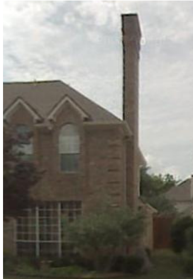
Figure 1. Pre-storm Chimney at Case Study A (Google Maps Street View)
